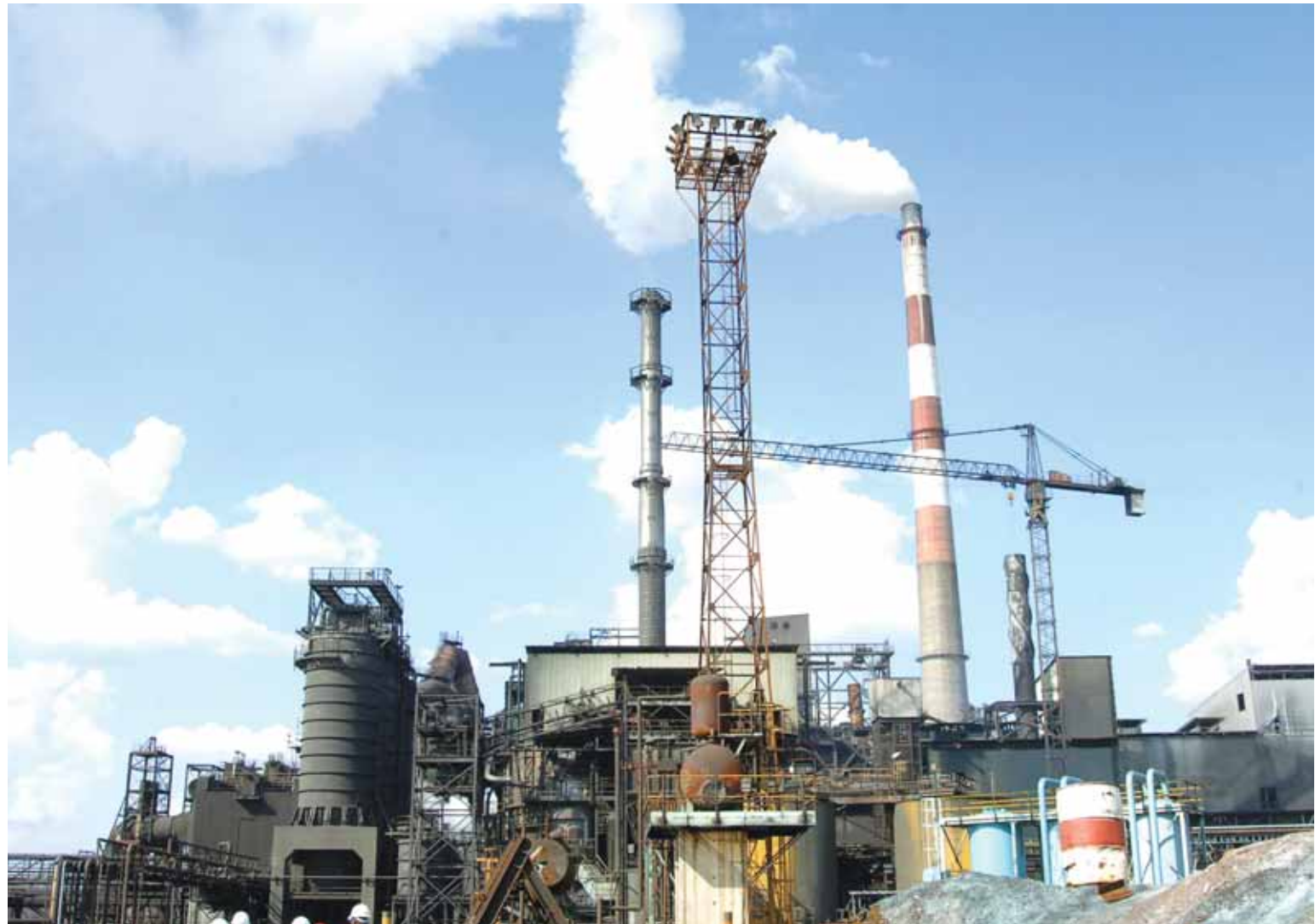
The iconic BCL mine chimney affectionately dubbed 'Chomela' embodies the town's rich industrial heritage and the spirited character that flourished during the golden age of mining.
