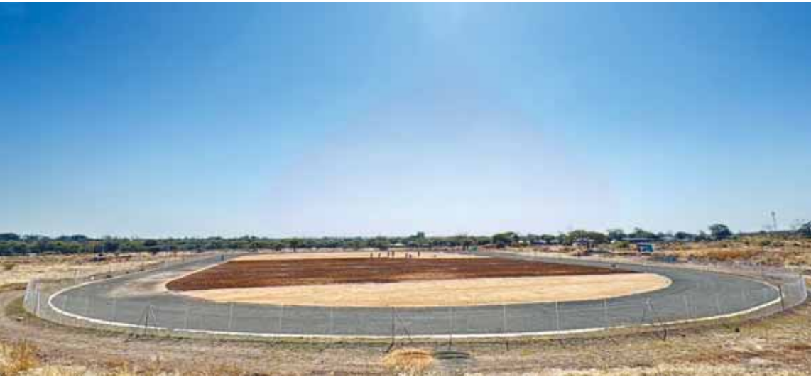
The base layers for the pitch and athletics track at Kasane Mini Stadium have been completed. Chobe District Council chairperson, Johane Chenjekwa said the facility was expected to transform the district’s tourism landscape by promoting sports and events tourism once construction was complete. Photos: Portia Keetile
