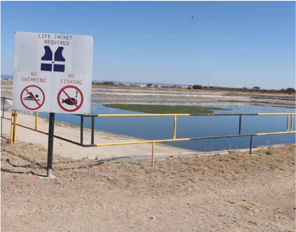
Malfunctioning sewer systems around Kanye are affecting village’s market place and for shoppers and traders, this is a daily life experience.
