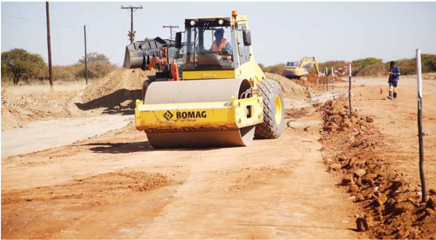
The ongoing construction of Modipane-Mabalane Road is at 32 per cent completion. When giving an overview, CPT Project Engineer, Mr Jacob Raphalane said recent rainfall caused the washing away of road layers and challenges in licensing of borrow pits delayed construction progress. The project that commenced on September 2024 is expected to be complete on April 2027. Photo: Phenyo Ramatu
