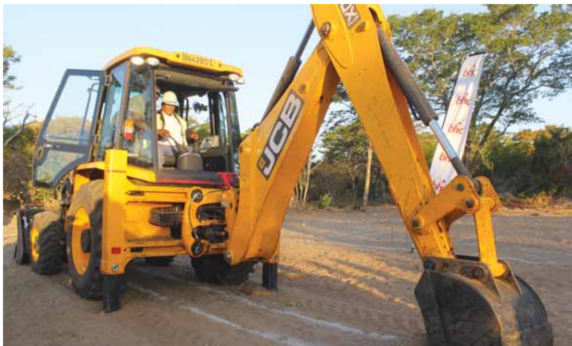
Minister Molale performing the ground breaking of the BHC housing project in Kazungula recently. The project comprises 176 standalone housing units and 36 high density housing. The first package is expected to be completed in August 2024. Photo: Portia Ikgopoleng
