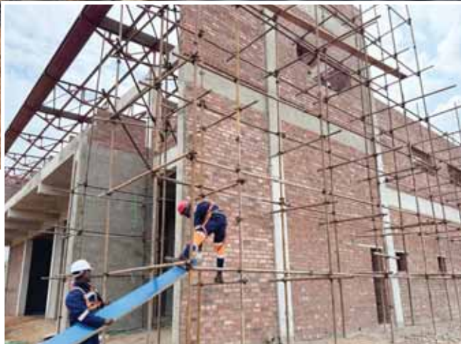
The Botswana Meat Commission Lobatse Tannery Revitalisation Project worth P218 million is anticipated to be complete by December. Colic Construction site agent, Mr Ermias Belay said the project was at 54 per cent, having completed civil works. The tannery consists of a hides processing area, chemical storage area, effluent treatment plant as well as an office block. Photo: Calviniah Kgauthe
