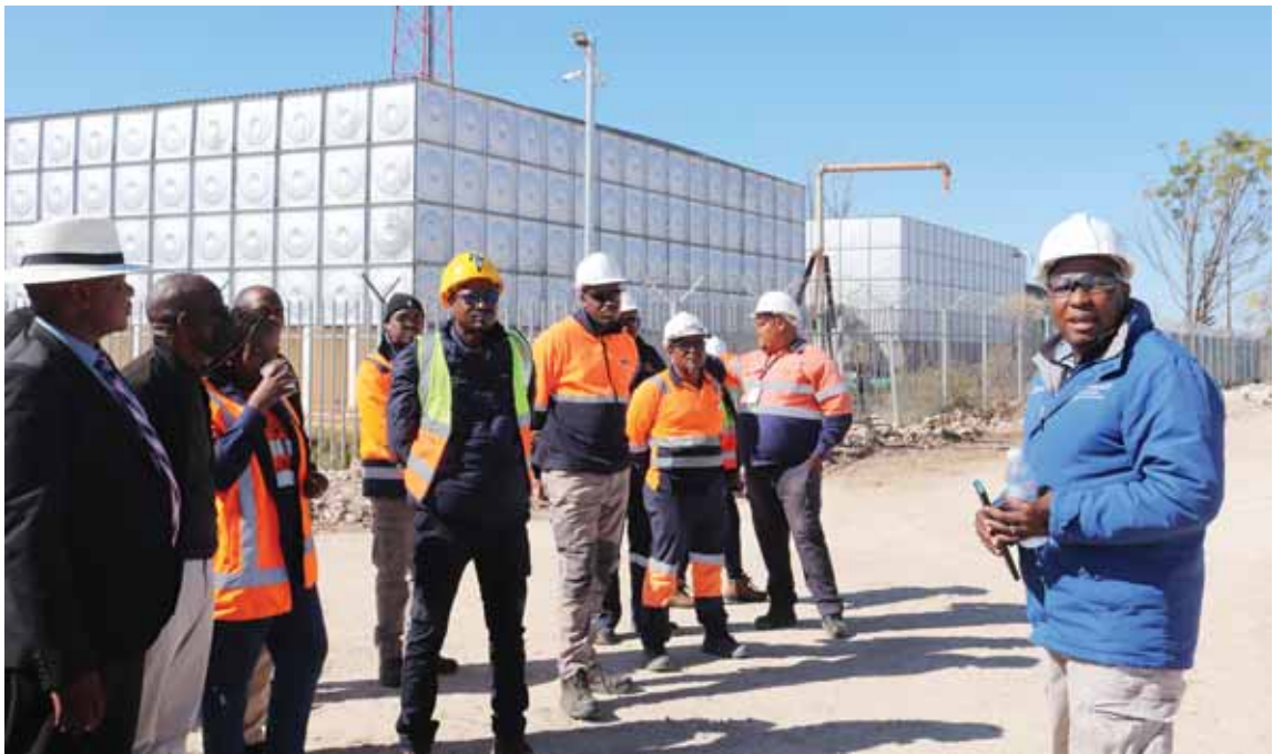
Jwaneng Mine project manager, Mr Letlhogonolo Ofithile (right) briefing the Jwaneng Mine general manager Mr Goitseone Gadifele and his delegation during a tour of the Magagarape Road construction project on Tuesday. The P74 million project is scheduled to be complete by end of August. Photo: Kehumile Moekejo
