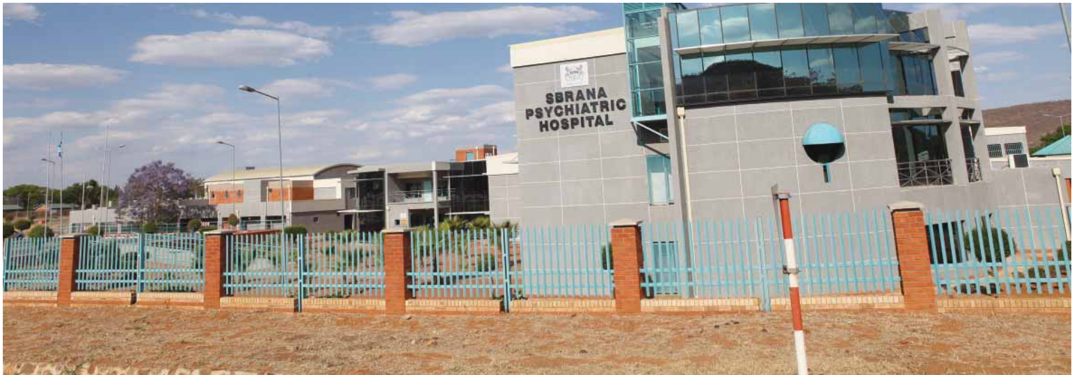
Recognising the need for long-term improvements, the Ministry of Health has developed a two-phased refurbishment programme to address infrastructure and maintenance challenges at Sbrana Psychiatric Hospital.
