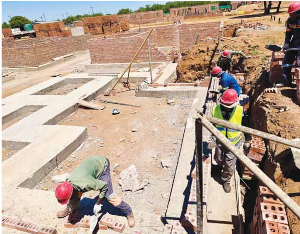
Upgrading of the Ramatlabama commercial border post project which started on May 5, is currently at 17 per cent completion rate. Botswana Unified Revenue Services Commissioner General Ms Jeanette Makgolo, said the benefit of improving borders was one of initiatives aimed at enhancing trade facilitation to streamline imports and exports. Photos: Calviniah Kgautlhe
