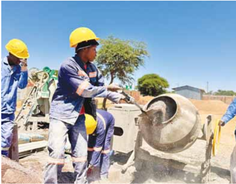
Construction workers on site at Ramatlabama Commercial Border Post.
