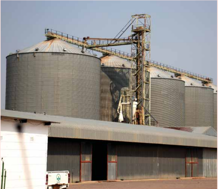
Botswana Agricultural Marketing Board acting strategy manager, Ms Ontlametse Ntshole said the P110 million refurbishment project of five Pitsane silos was expected to start in the near future. Photo: Aobakwe Molefhi
