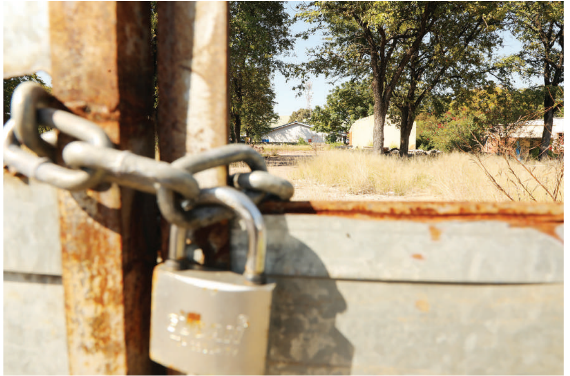
Francistown Central Market demolished years ago after a court ordered the eviction of illegal occupants to make way for redevelopment. Francistown mayor, Mr Gaone Majere said the developer would begin work next month. Photo: Ogopoleng Kgomoethata
