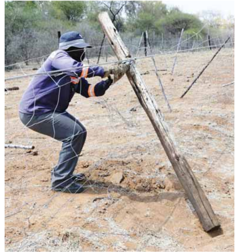
Ministry of Agriculture employee repairing part of the Matsiloje and Dikgathong fence on Monday. Photo: Gaseitsewe Moruakgomo
