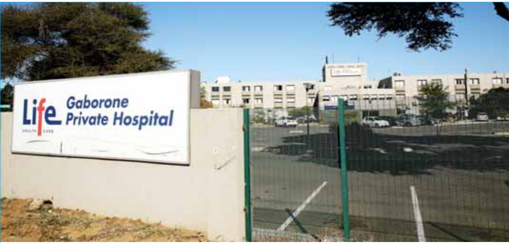
Gaborone Private Hospital is one of the modern healthcare facilities that have expanded access to specialised medical services in the country.
