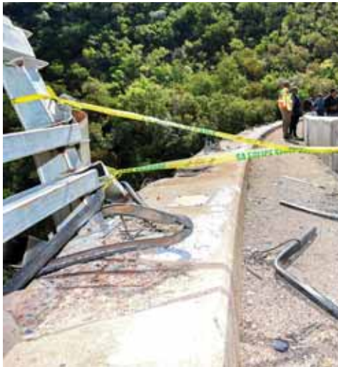
The spot where the bus plunged off Mamatlakala Bridge, catching flames as it hit a rocky ground
