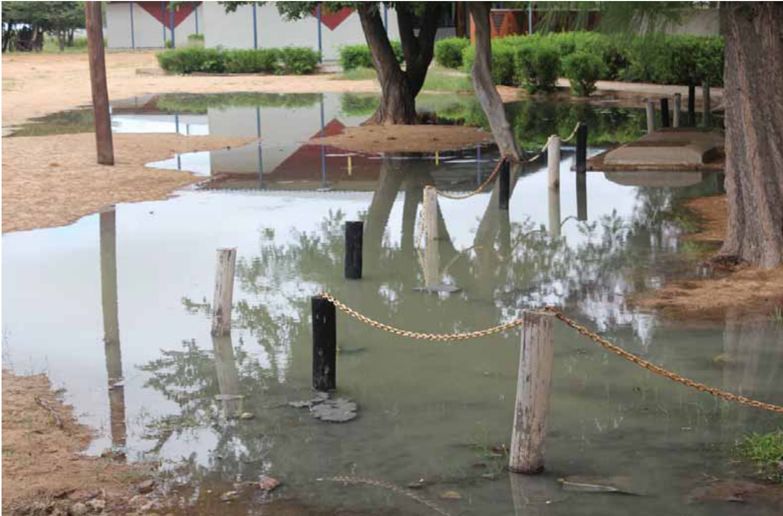
An over spiling sewage at one of the schools in Botswana. Mogoditshane/Thamaga District Council chairperson, Mr Molatedi Selala, has proposed the immediate closure of Thamaga Junior Secondary School over a persistent sewerage problem he considers a serious public health crisis.
