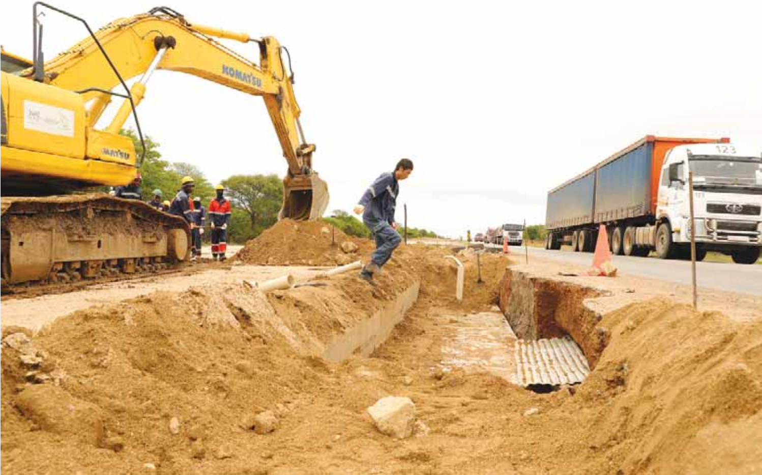
The A3 Road re-construction project has been unbundled into strategic sections to allow construction companies to work simultaneously. Okavango Africa Consortium representative, Mr Boyce Mohutsiwa said section two and three of the Francistown-Nata corridor, was at 34 per cent against the targeted 39 per cent, noting that the company would take advantage of the coming dry spell to cover lost time.
