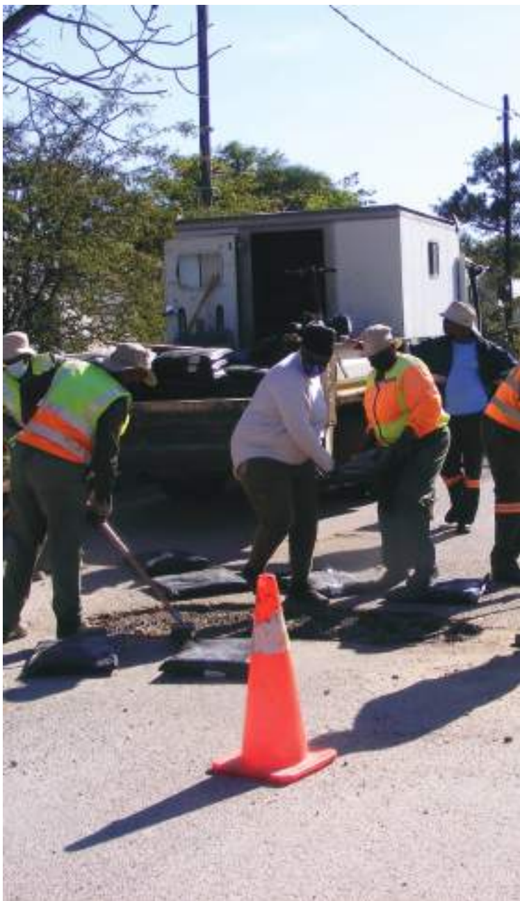
The City of Francistown Council requires approximately P12 million for pothole patching and related maintenance work, while an estimated P335 million is required for comprehensive road reconstruction, upgrading, reclamation, and storm water drainage improvements along critical road sections. The mayor, Mr Gaone Majere said the council had already sourced 7 000 bags of cold asphalt premix, sufficient to patch approximately 3.500M metre square of potholes. Photo: Thamani Shabani
