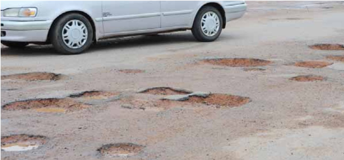
Residents of Francistown have joined the city council in a 14-day community drive to patch potholes across the city’s damaged road network.
