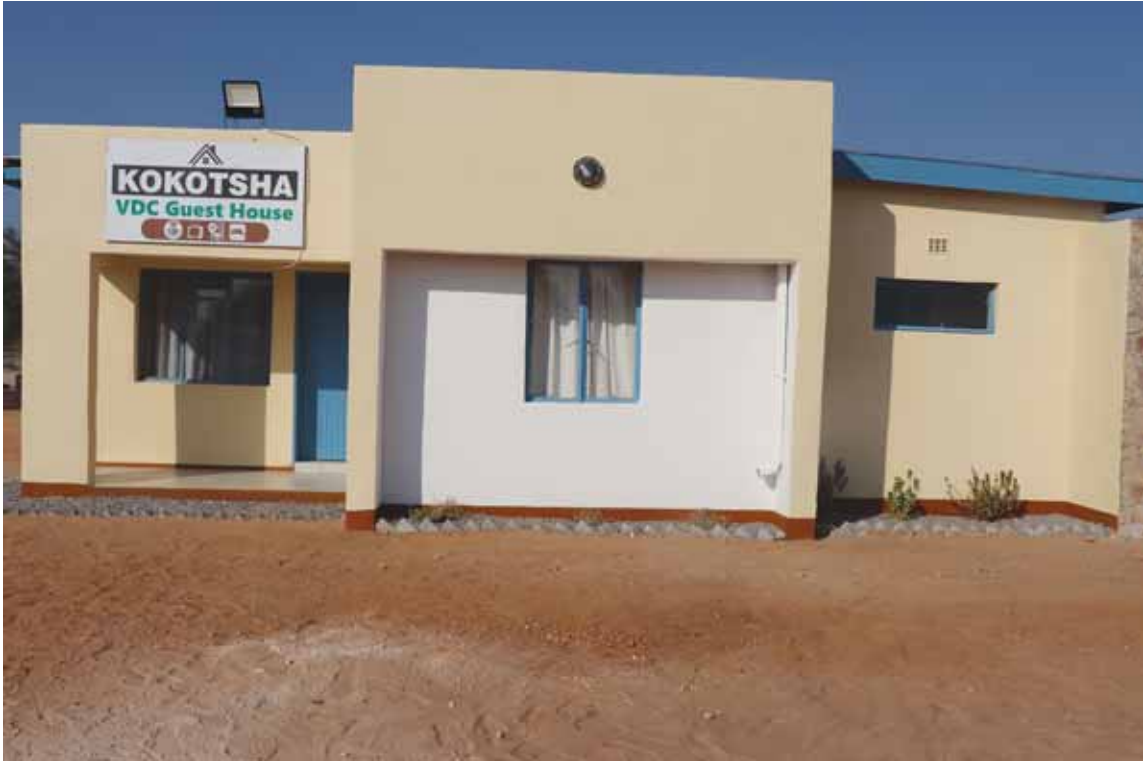
A long-cherished community dream has become a reality with the official opening of the newly expanded and renovated Kokotsha VDC Guest House. Once a modest vision, the facility now stands as a symbol of community-driven development, promoting hospitality, economic empowerment and self-reliance while creating new opportunities for tourism growth. Photo: Naomi Leepile
