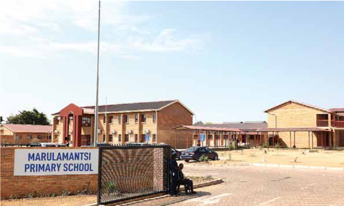
Marulamantsi Primary School is currently embarking on a project to construct an onsite swimming pool.
