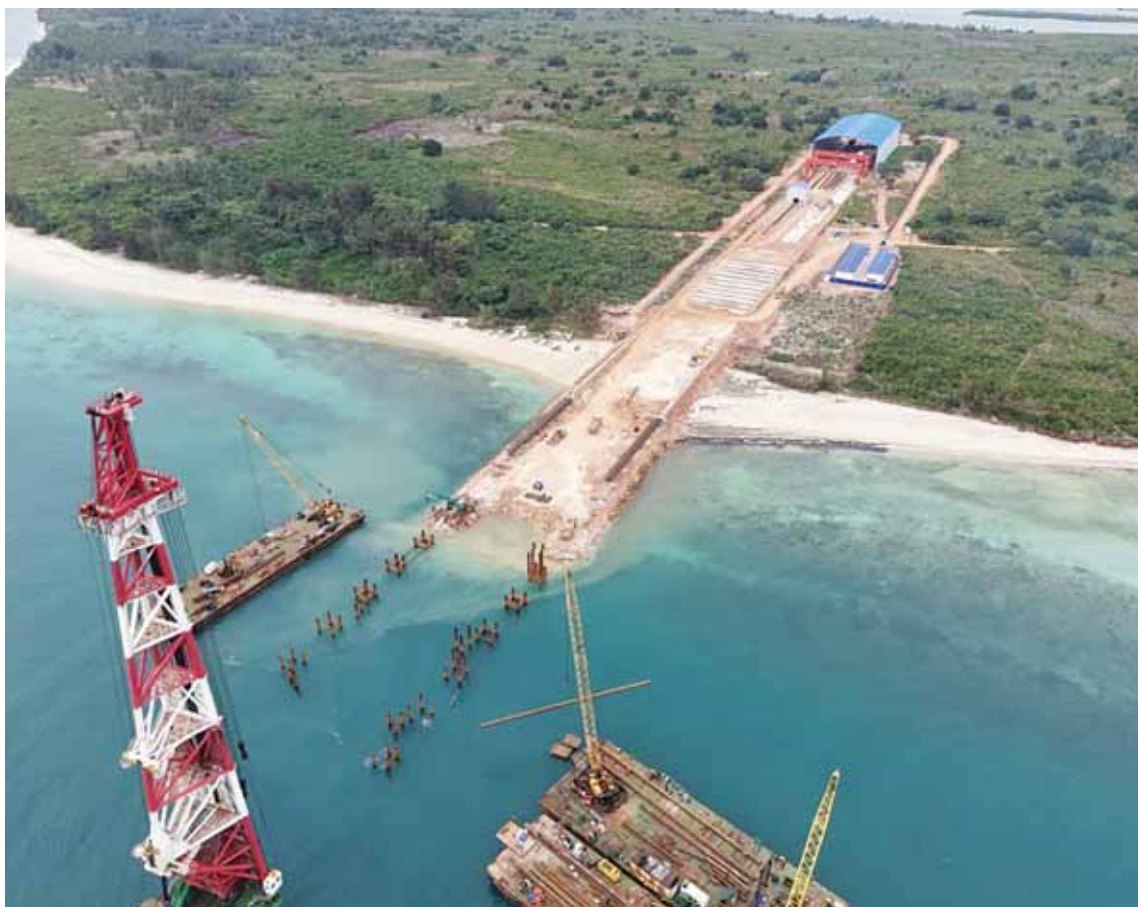
ZANZIBAR - A steel pipe plant at the construction site of the Zanzibar Mangapwani new port project in Tanzania. The project has employed 500 people, with local workers accounting for around 80 per cent. Photo: Xinhua
